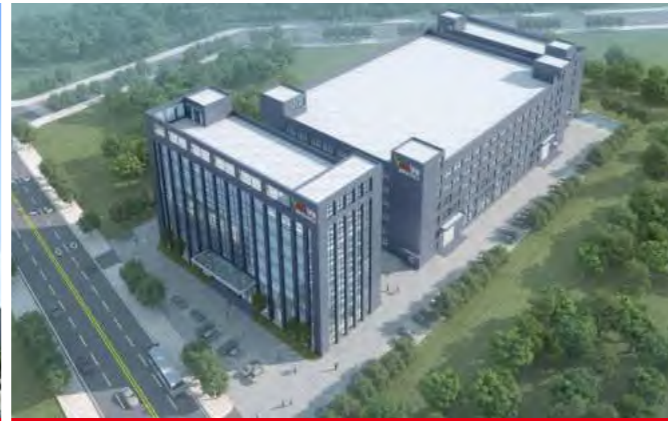
伊发5G智慧数字化工业园·乐清湾港区一期 YIFA 5G Intelligent Digital Industrial Park Phase I of Yueqing Bay Port Area
